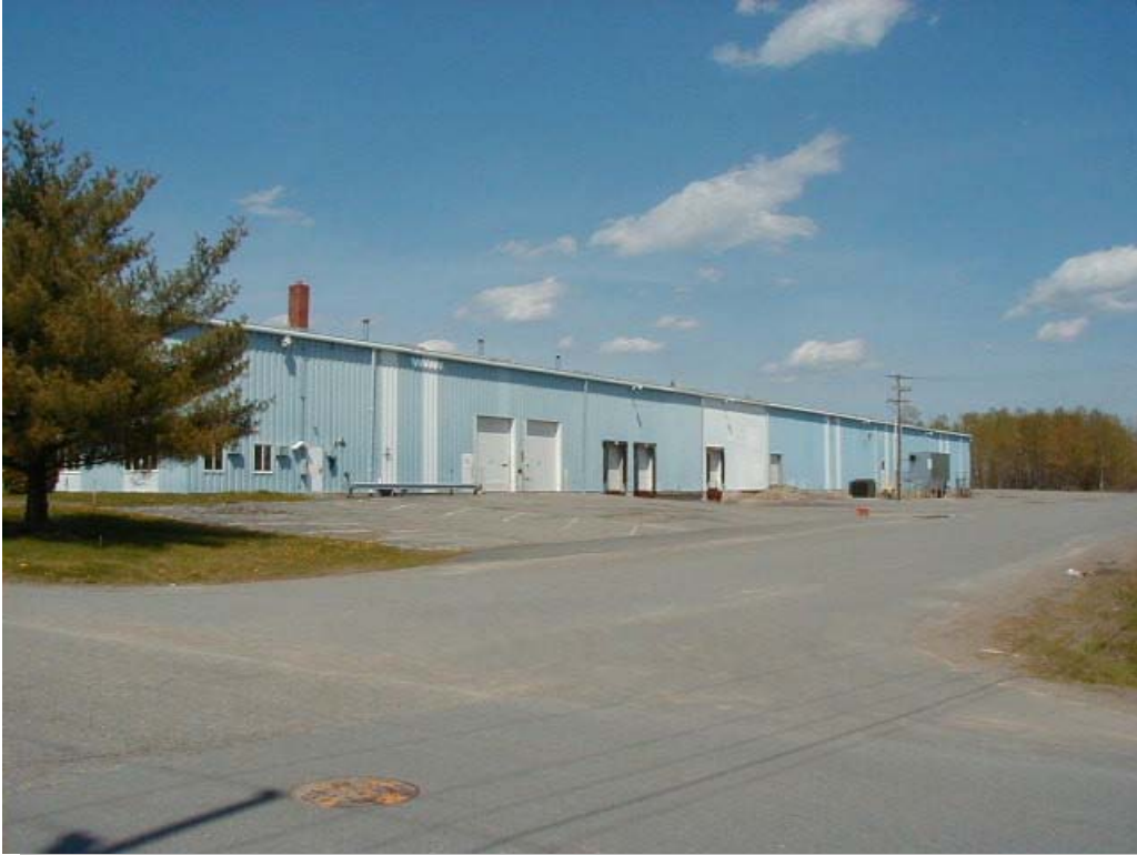
Exterior: South Side
